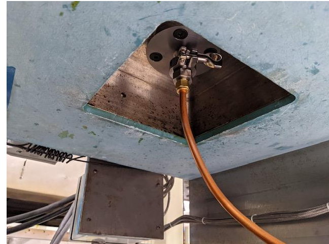
Bottom resin injection setup
